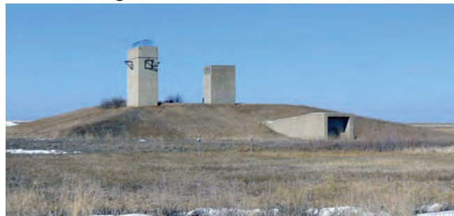
RSL 1 RLOB entrance tunnel and stacks
